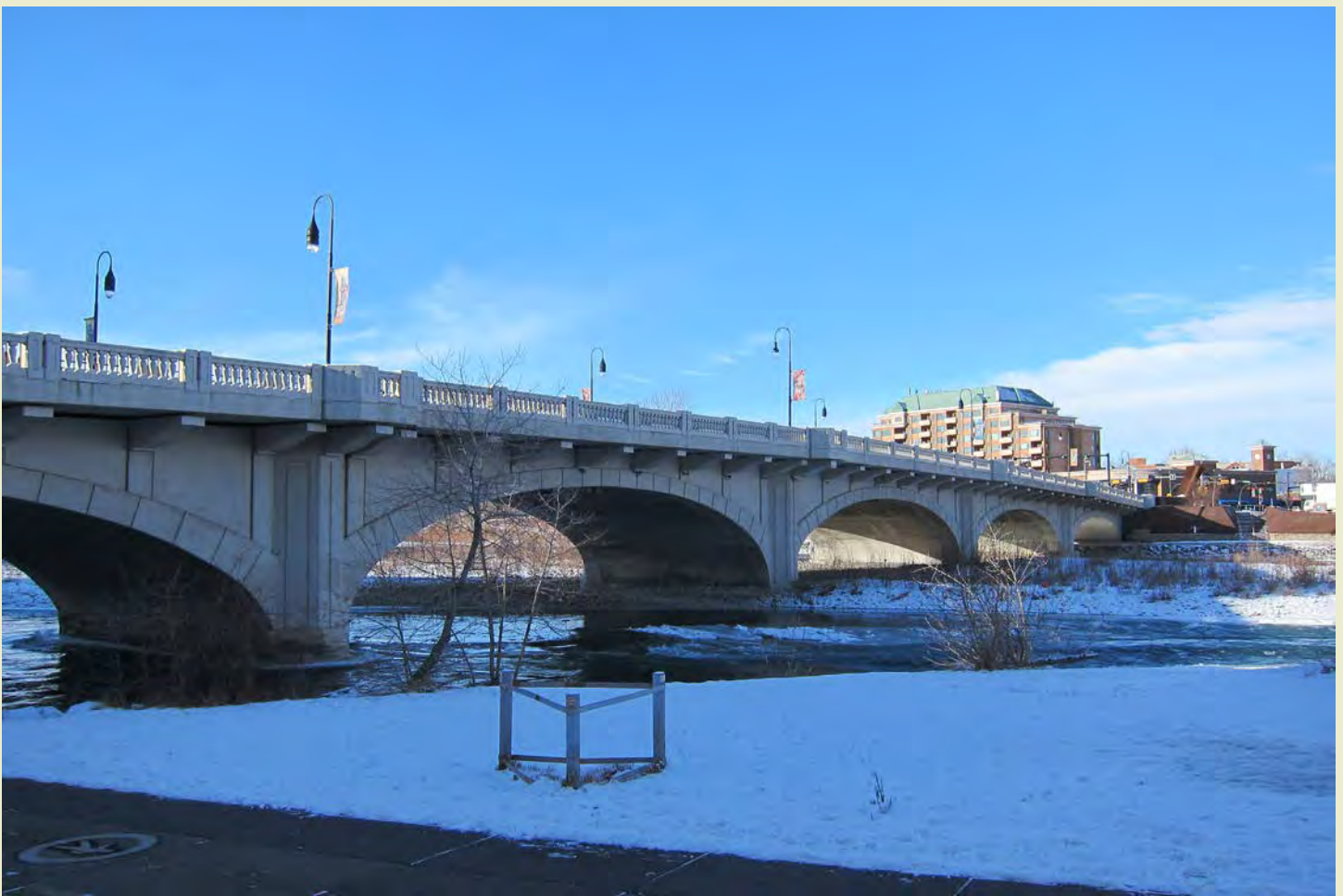
Louise (Hillhurst) Bridge looking from the southeast
