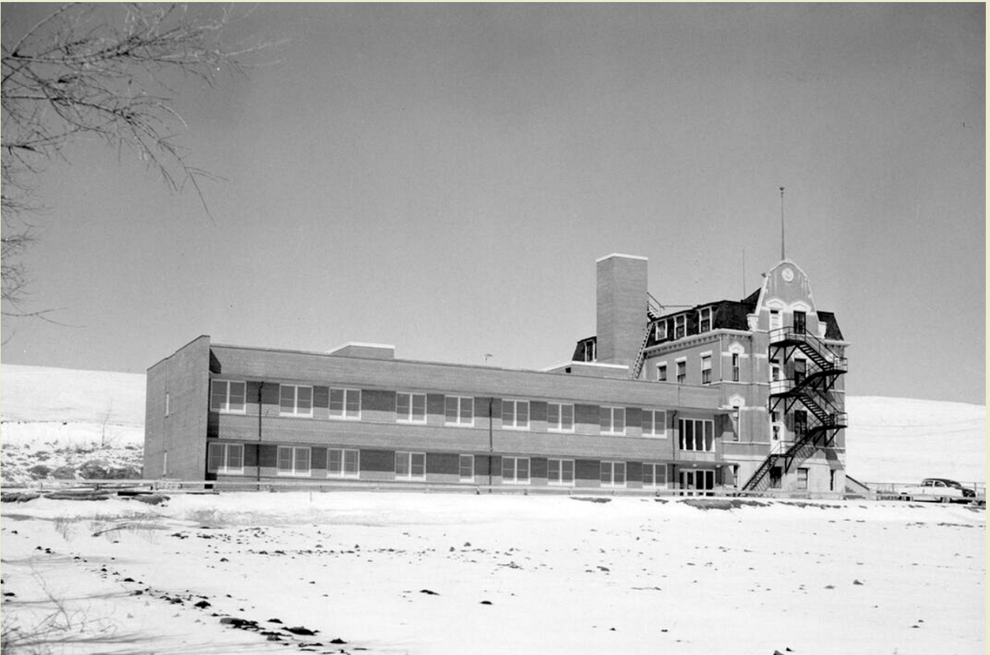
Grace Maternity hospital, 1954, with new west wing [Photography by Jack De Lorme, Credits: Glenbow Archives na-5600-7431a]
