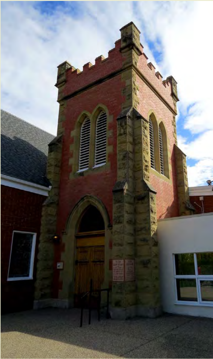
St. Barnabas's Church Tower
