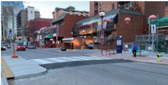
Photo of Continuous Sidewalk with bump outs on 3 Ave SE in Chinatown, Calgary.
