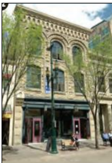
Figure 3. The Ashdown Block on Stephen's Avenue. Built in 1891 from sandstone taken from Orr's north bank quarry below East Crescent Heights.
