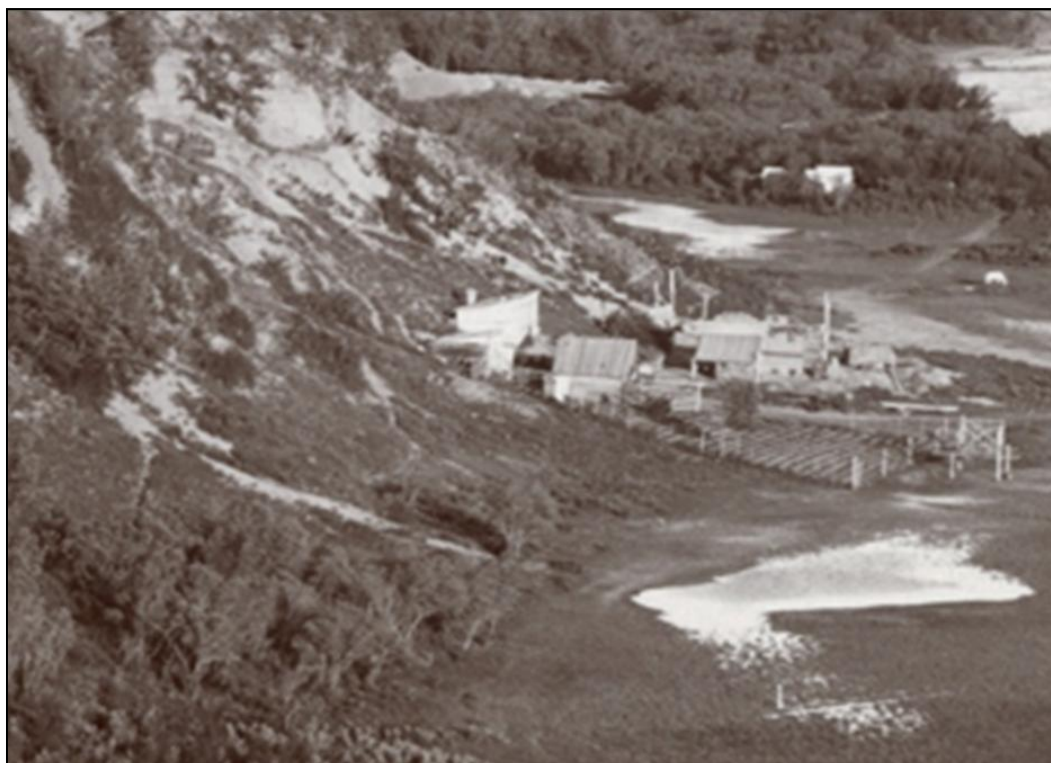
Figure 10. A zoom-in of figure 9 photo of buildings located at base of slope with a horizontal bench cut further up the slope. Further east, beyond the first trees, there is another light-coloured debris slope that may indicate quarrying above.
