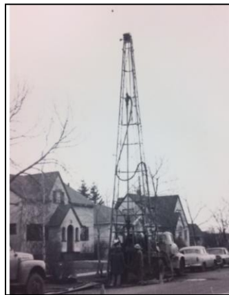
Figure D8. 1959 Geotechnical Drilling on Alexander Crescent. The same houses are still there in 2022. The City of Calgary Archives (copyright; cannot be reproduced without obtaining permission of City Archives).
