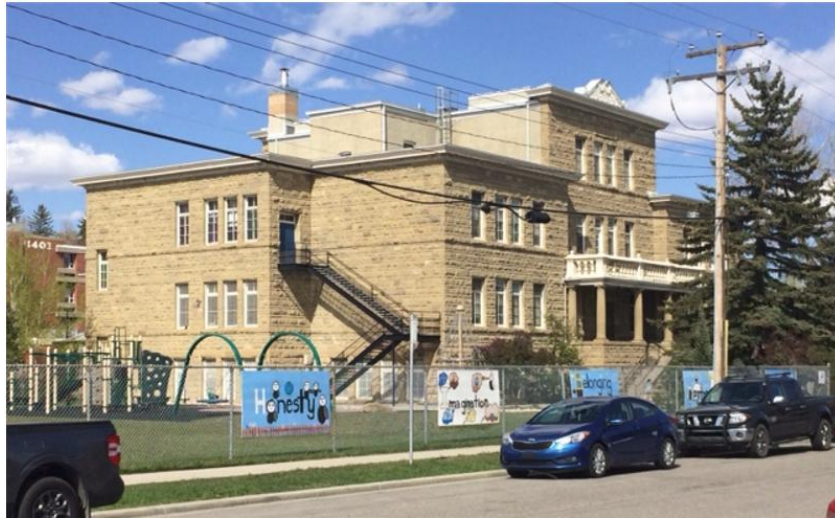
Figure 8. Hillhurst School. Built in 1912, it was one of the last of the sandstone schools to be built. The sandstone blocks are of uniform size in comparison to the 1890 courthouse.
