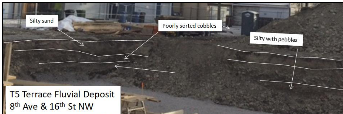
Figure A2. A 2022 photo of a construction site located at 8th Ave. & 16th St. N.W., just south of the base of the escarpment. The cobbles and pebbles are river gravels associated with the T5 River Terrace. The shallow silty sand layer may be glacial lake sediments that were eroded from the adjacent escarpment.
